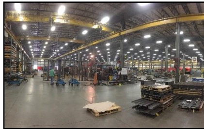
Before: 32 watt T8 Fluorescent lamps 5000K
